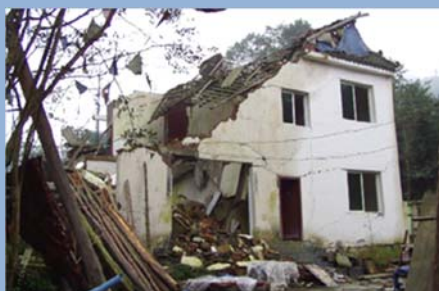
Collapsed brick masonry structure (Sichuan)
