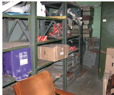
Shelves containing medicines etc. without anchorage
