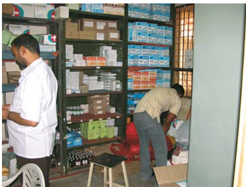
Shelves containing medicines etc. without anchorage
