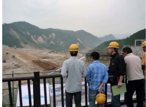
Photo 4-34 Observation at the Isawa Dam construction site [Isawa Dam Construction Office, MLIT]
