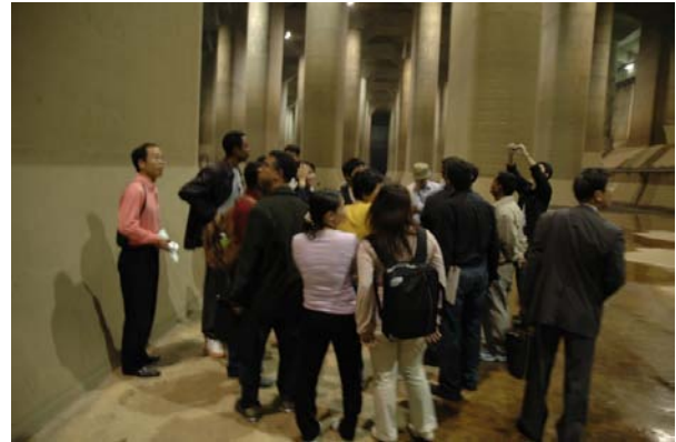
Photo 4-11 Inside the surge tank of the Metropolitan Diversion Channel [Edo River Work Office, MLIT]
