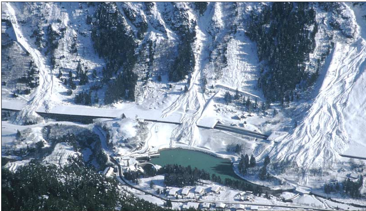
Figure 4.8 Due to many avalanche galleries, many avalanche-prone roads and railways could still be kept open in the 1999 catastrophic avalanche situation in Switzerland. The picture shows the Gotthard highway in February 1999
