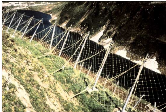
Figure 4.3 Snow nets stabilise the snow in a potential avalanche starting zone
