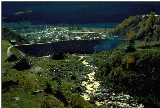
Figure 4.4 Avalanche retaining dam in Trun, Canton Grisons, Switzerland
