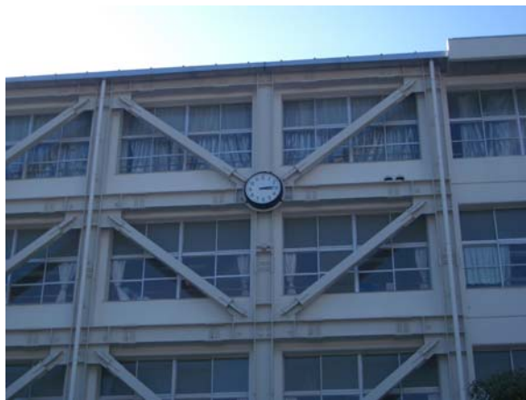
After retrofitting (exterior)
