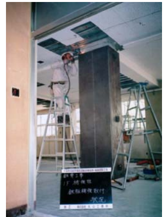
Steel jacket column reinforcement
