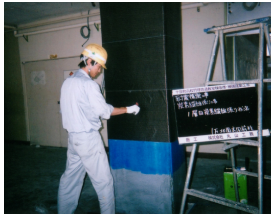
Carbon fiber jacket column reinforcement
