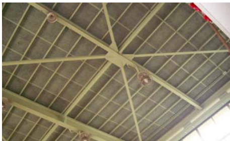
Bracings along the roof Detail
