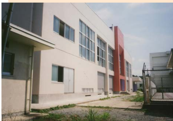
After retrofit (outside view)
