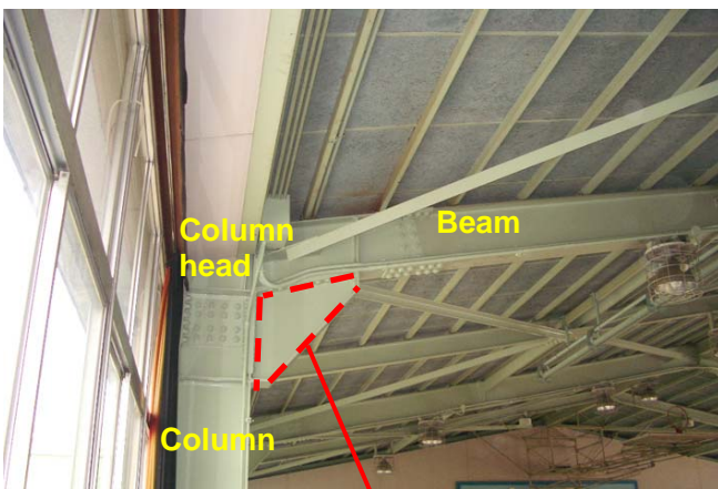
Reinforce column-beam joint by installing rib-plates
