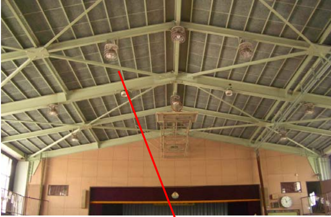
Bracings along the roof
