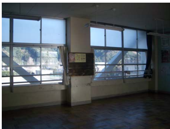
After retrofitting (interior)
