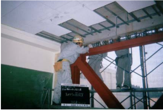
Installing a steel bracing
