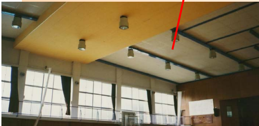
After retrofit (inside view)
