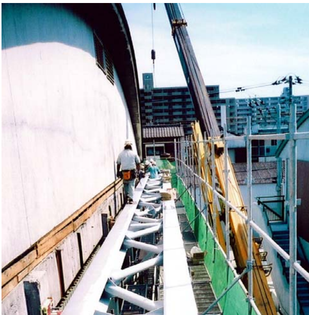
Erection of steel frame
