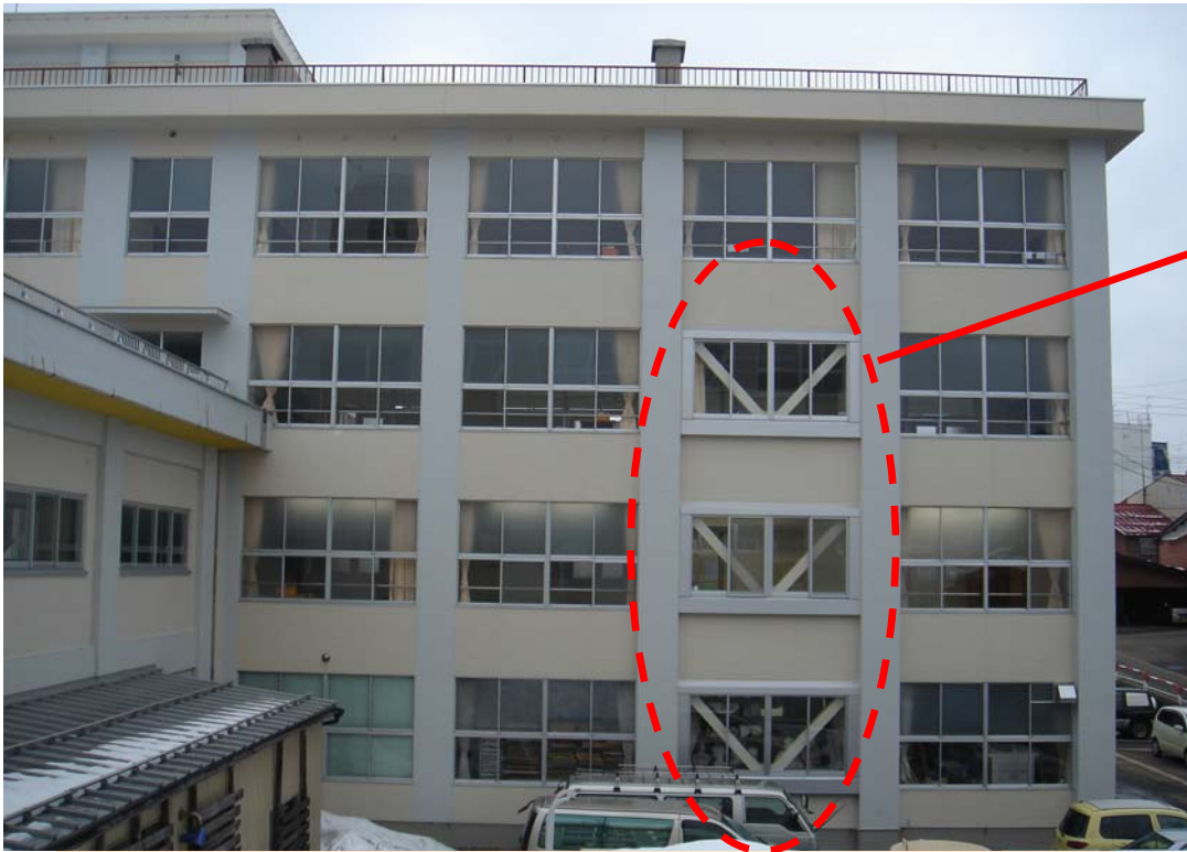
After retrofit (outside view)
