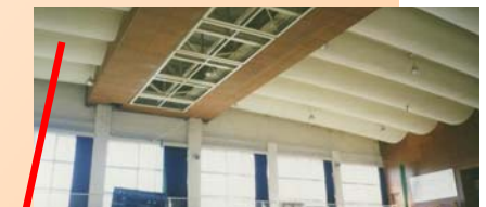
Before retrofit (inside view)
