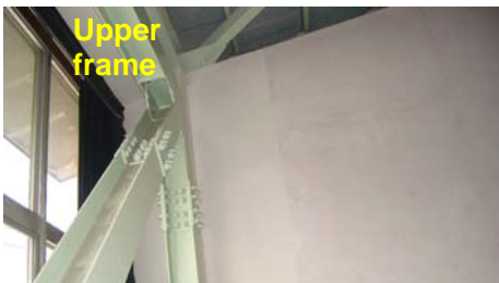
Steel bracings Detail-1
