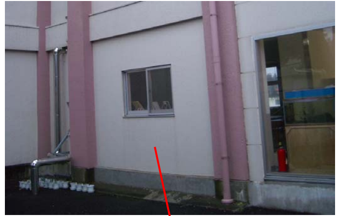
Installed shear wall
