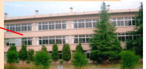
Before retrofit (outside view)
