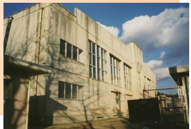
Before retrofit (outside view)
