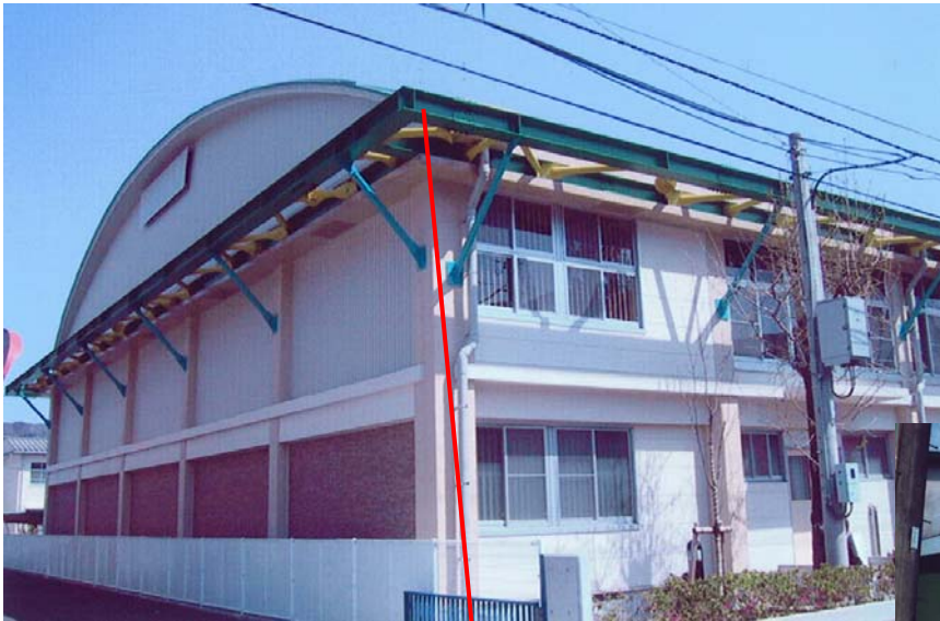
After retrofitting (exterior)
