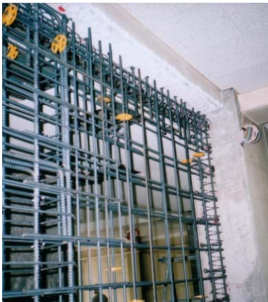
Adding the seismic shear wall
