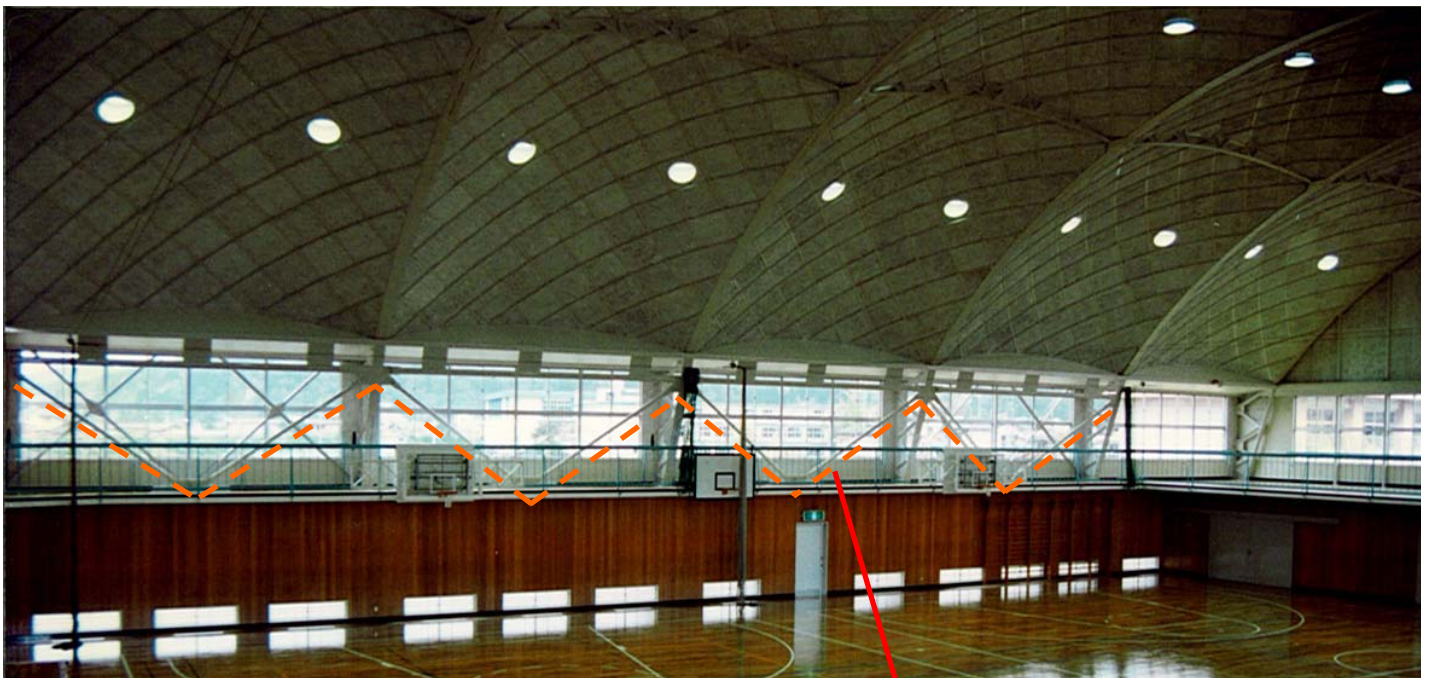
After retrofit (inside view)
