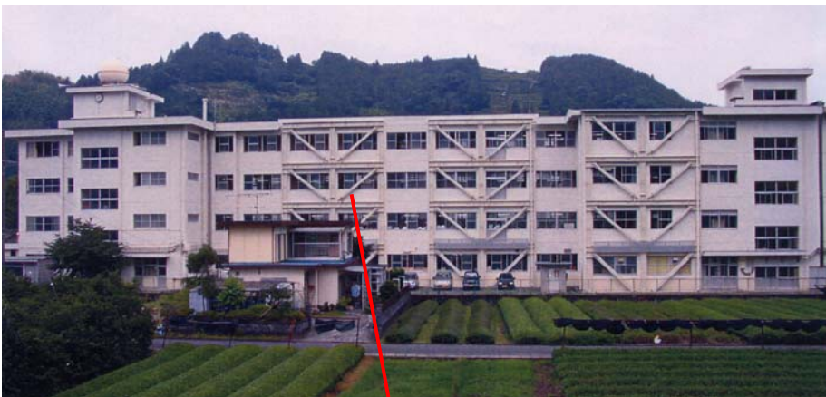
After retrofitting (exterior)
