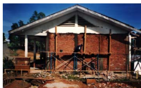
School building undergoing structural reinforcement
