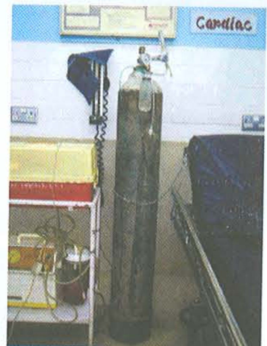
Hooking 8:8 Hooking the cylinder with a chain can save the cylinder from falling.
