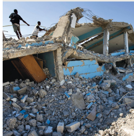
It is not earthquakes that kill people but the buildings collapsing on them. (UN Photo/Logan Abassi)
