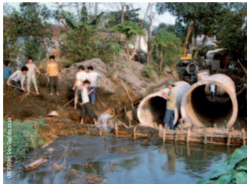
Improving water and sanitation infrastructure in Viet Nam.
