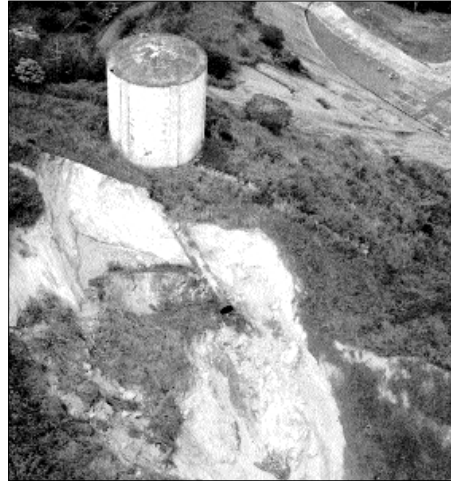
Landslide at storage tank.
