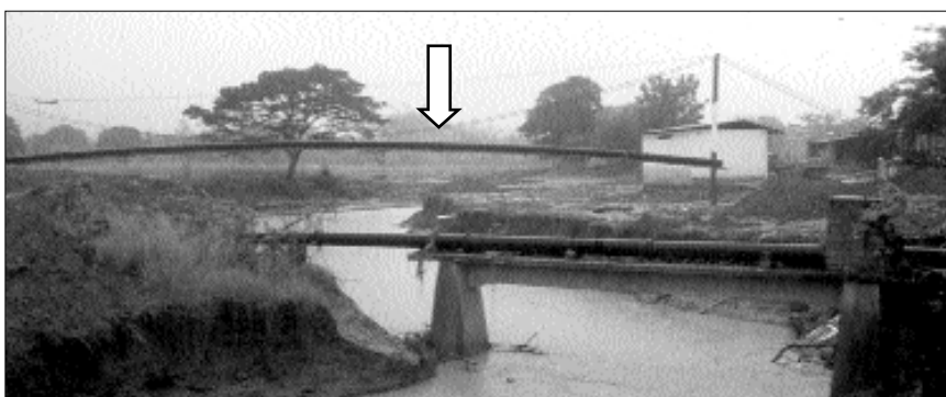
This photograph shows the effects of flooding during El Niño in Ecuador in 1999. The construction of a river overpass is a mitigation measure for piping.
