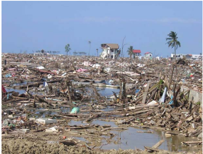
Waste and debris in Banda Aceh
