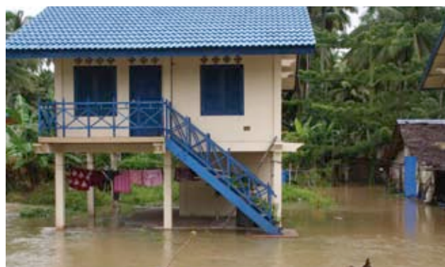
Reconstruction: earthquake resistant and flood proof houses within a GRC project in Indonesia after the Tsunami of 2004. Photo: GRC 2008
