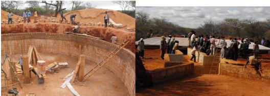
Photos: Burduras, Kukub, Burashin, Mandera, Kenya - underground tanks under construction and upon completion
