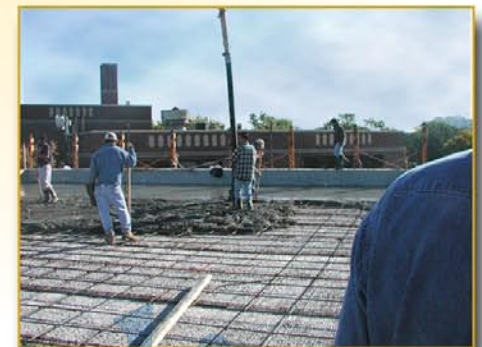
Pouring the 4-inch concrete roof deck.
