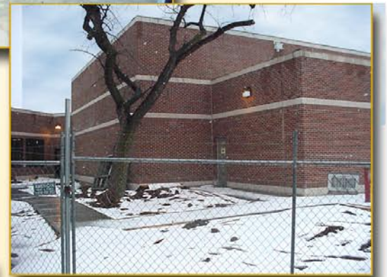
Exterior of Park Elementary multipurpose shelter.
