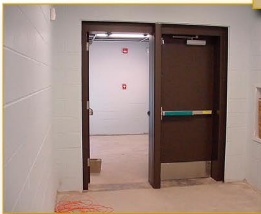
Perimeter door with six-point connection at McCollom Elementary. Like the windows, all perimeter doors in the shelter are also welded to embedded steel plates and have six points of connection.
