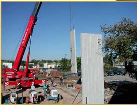
Crane placing precast concrete wall panels.
