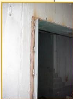
Perimeter door with six-point connection at McCollom Elementary. Like the windows, all perimeter doors in the shelter are also welded to embedded steel plates and have six points of connection.
