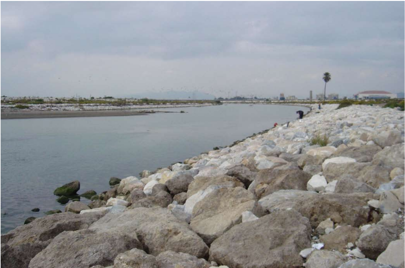
River Guadalhorce flood prevention levee, Spain, soon after completion in 2003. A double levee construction was made to avoid a repeat of the devastating 1989 floods.
