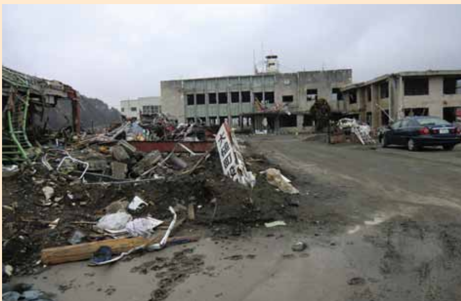
FIGURE 5: Otsuchi city hall after the tsunami struck
