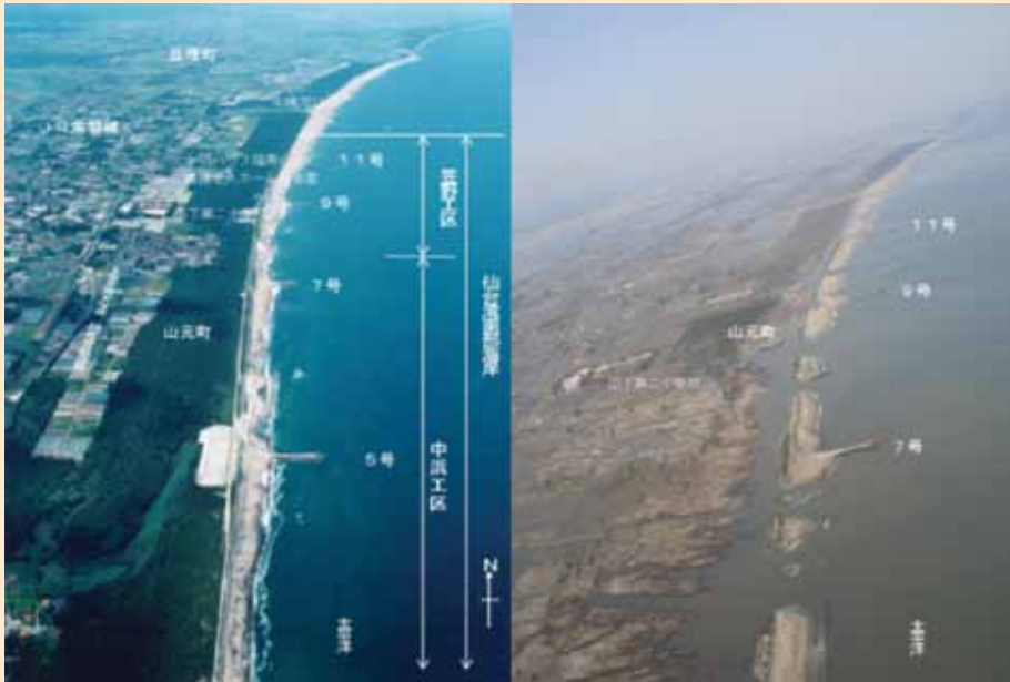
FIGURE 4: Dikes in Sendai before and after the tsunami of March 11, 2011
