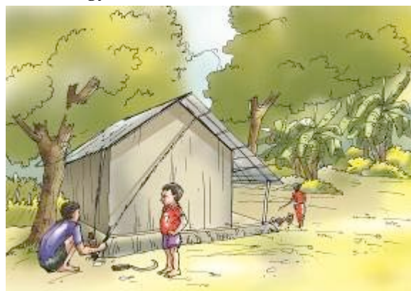
Tying roof of house with veranda and mud walls with wooden pegs fixed on the ground
