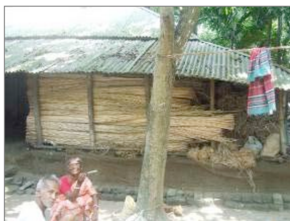
Laying bricks in a row to prevent damage to plinth area from rain water falling from roof
