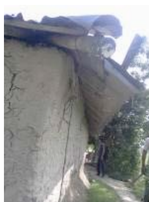
Tying roof of house with veranda and mud walls with wooden pegs fixed on the ground
