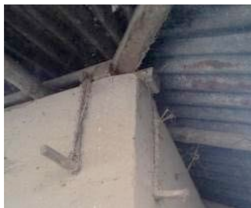
Tying roof of house with veranda and mud walls with wooden pegs affixed to the ground
