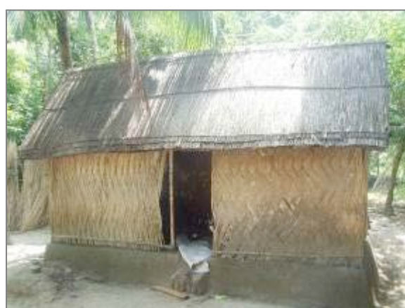
Building houses using jute stalks to reduce damage due to hazards
