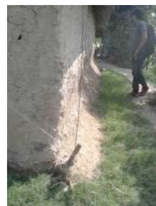
Tying roof of house with veranda and mud walls with wooden pegs fixed on the ground
