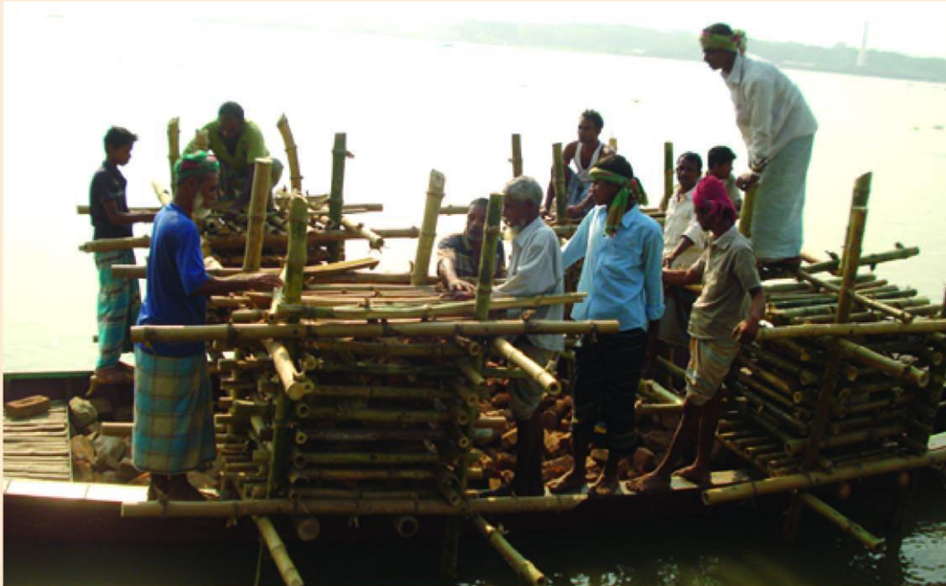
Mitigate River Erosion
