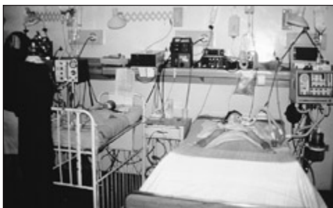
The equipment in an intensive-care unit should be secured against toppling and sliding during earthquakes. (Photo PAHO)
