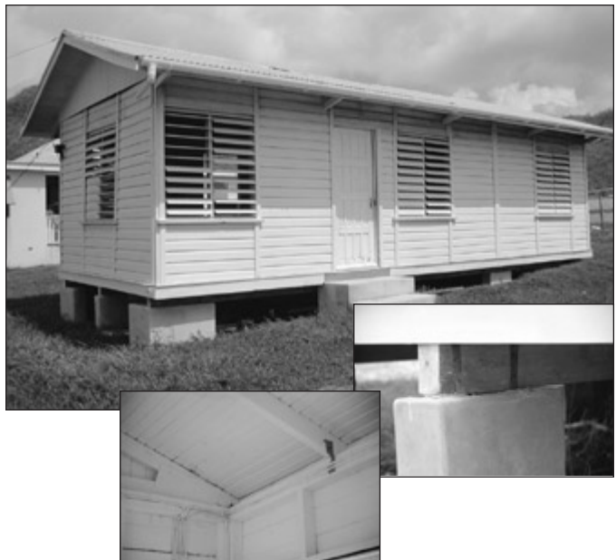
This rural clinic, although built of lightweight materials, survived a severe hurricane because of adequate connections at the bases and the roof. (Photo Tony Gibbs)
