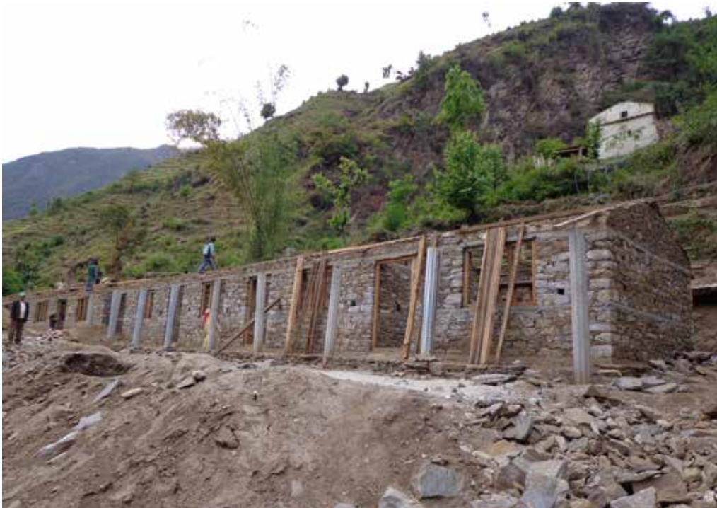
Picture 8: The re-construction of Lamabagar Primary School (April 2014) (Mission East, 2014)
