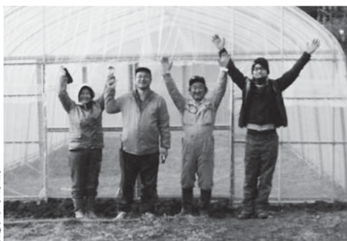
Finishing the construction of a greenhouse for seedling nurseries in Hirota-cho, Rikuzenataka City. Second from right is Mr. Chuichi Shida, Chairman, Hirota Horticulture Association. (28 February 2014)
