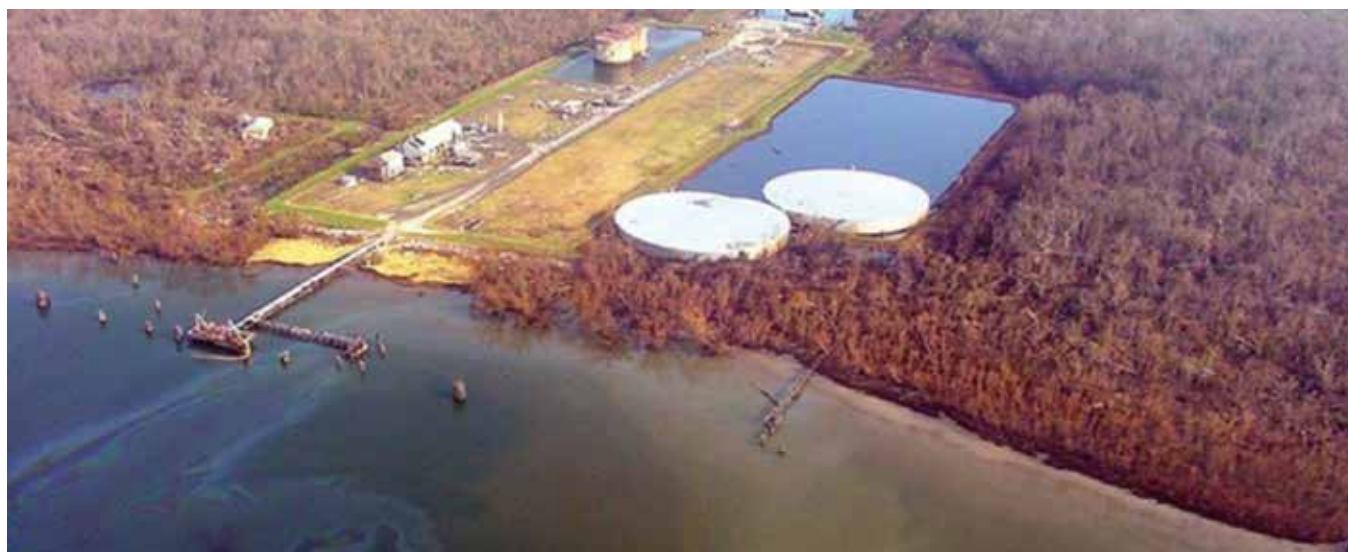
Oil spill in Louisiana due to Hurricane Katrina impact.
