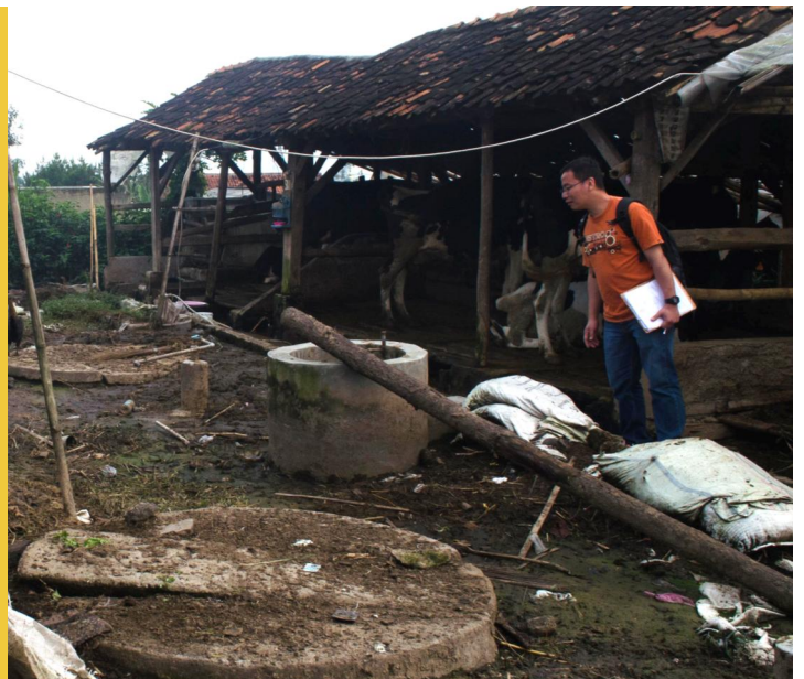
RDI Team observing a biogas inlet outside a barn at Cibodas Village
