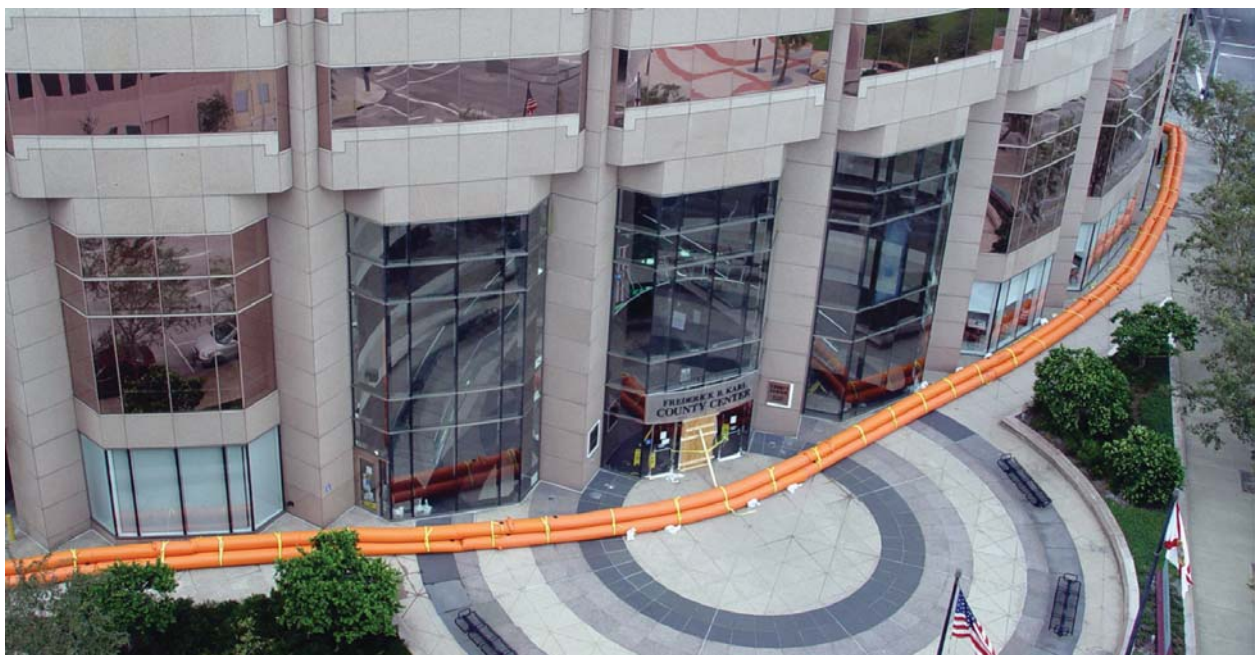
Example picture of Tiger Dams set up around an office building.
