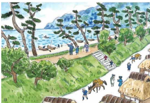
Hiromura Embankment built by Hamaguchi Goryo
