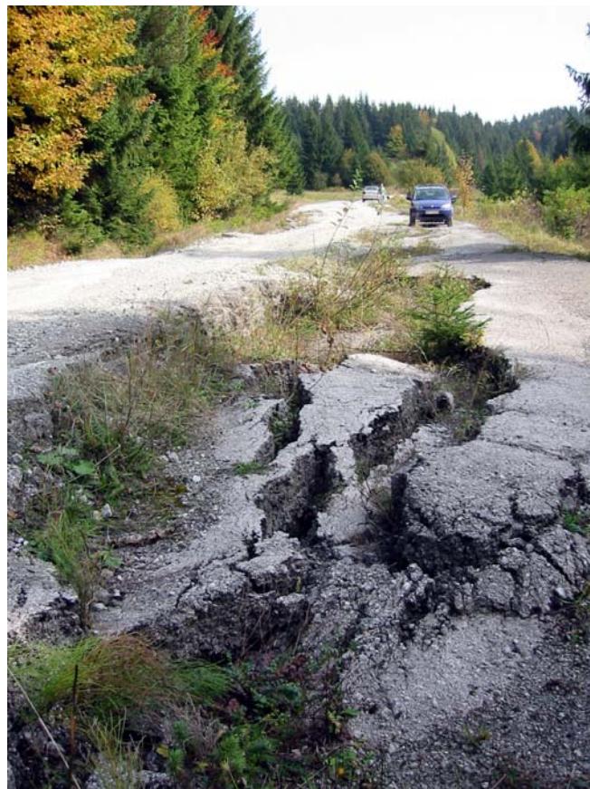
Figure 3: An old road destroyed by landslide close to Harvelka village, northern Slovakia (Photo by R. Jelínek)
