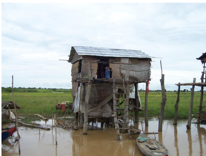
Figure 4. House in Cambodia
