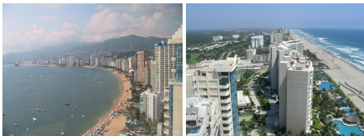
Figure 5. Aerial pictures of Acapulco nowadays. Bay of Santa Lucia (left) and Beach Diamante (right)
