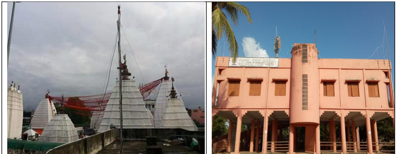
Figure 17 Lightning Safe Grid at Babadham Jharkhand and Safe Cyclone Shelter at Odisha
