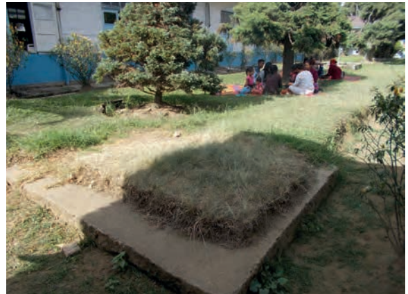
V4- Cover septic tank
