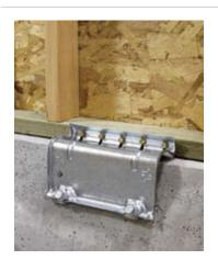
UFP Installation, Anchoring the Mudsill to the Foundation (see page 11)
