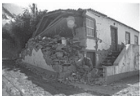
Figure 8.8. Collapse of external rubble masonry walls in kindergarten in Salão
