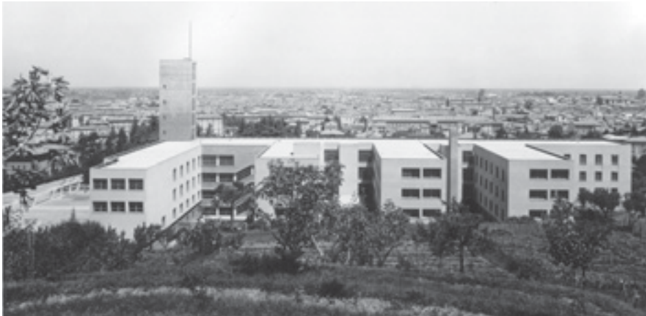
Figure 14.3. The Faculty of Engineering at the University of Bologna
