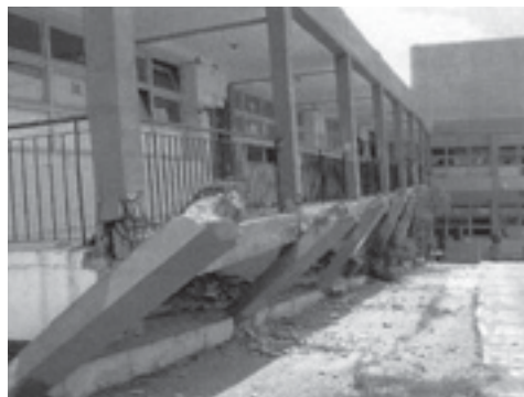
Figure 1.4. Collapse of first floor due to column failure
