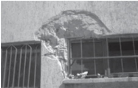
Figure A4.7. Typical confinement detail of a column in building C-13-09
