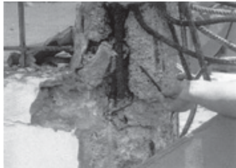
Figure 1.4. Collapse of first floor due to column failure
