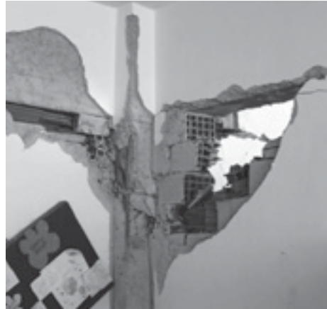
Figure A4.7. Typical confinement detail of a column in building C-13-09
