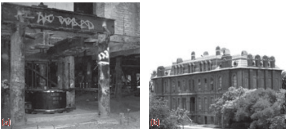
Figure 14.8. (a) Exterior view of excavation, showing temporary supports and scale of the project, Berkeley University Campus (b) Oldest building still standing on the campus, South Hall, Berkeley University Campus
