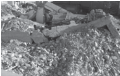
Figure 3.1. Rubble stones, reinforced-concrete kerb in the ruins of the San Giuliano primary school
