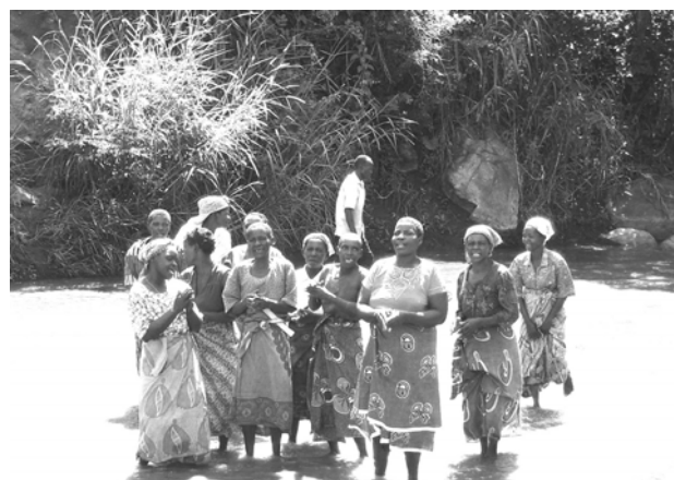
Dam Building Project under FFA in Balaka District
