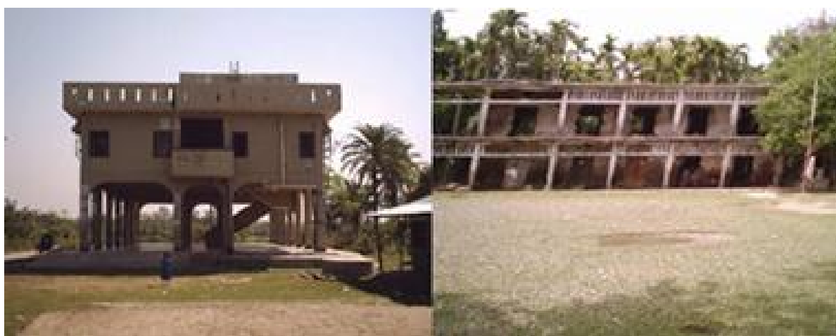
Figure 1.2: Cyclone shelter in good condition (left); needs repairing (right) [photo: CEGIS]
