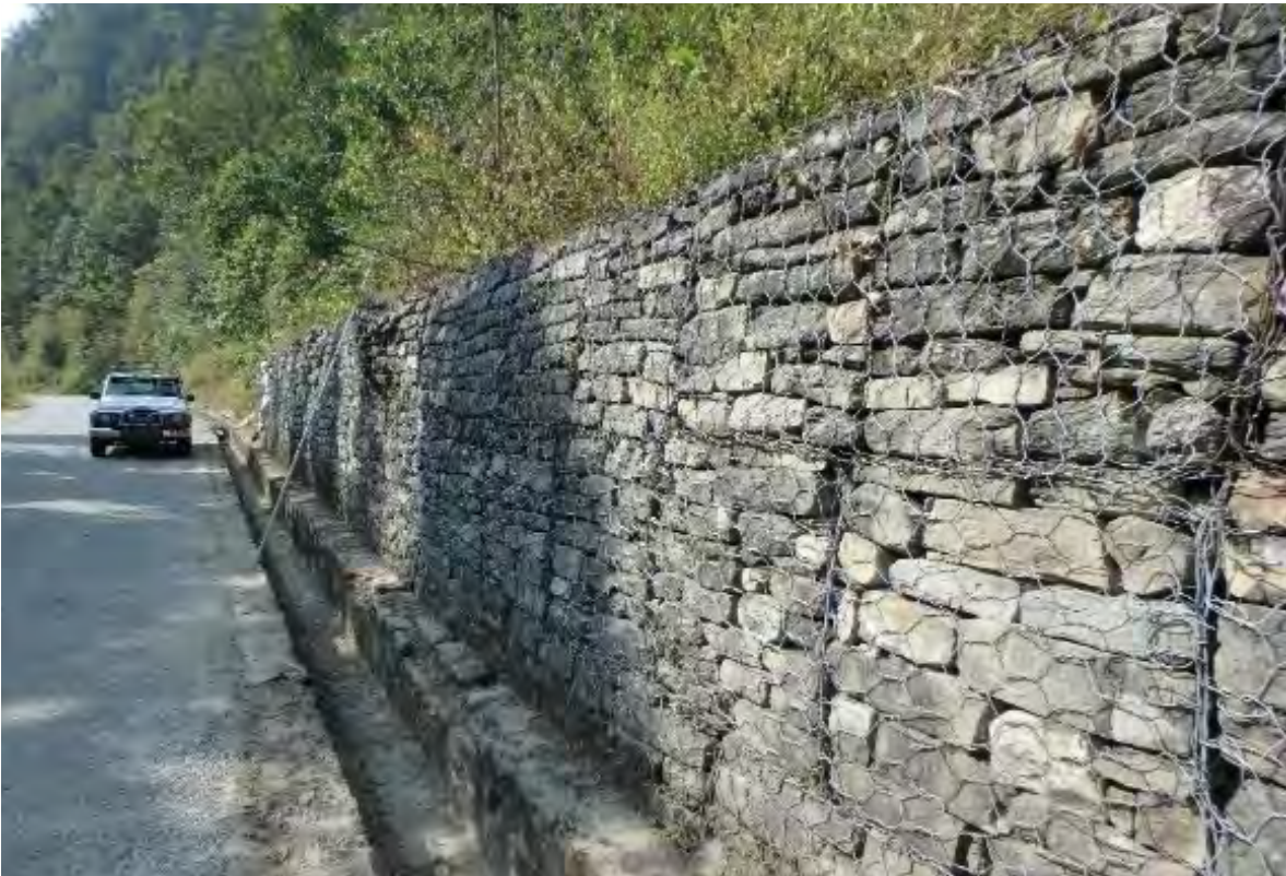
Figure 1: Gabion Retaining Wall for Road (Photo by Dr. Nakazawa)
