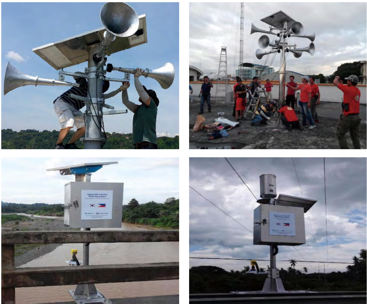
Figure 4. Installing the flood warning system in the Philippines. Photo credit: NDMI.
