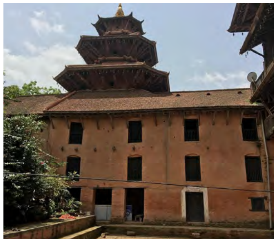
Figure 5. The building as the pilot project using the Power Coating (inside only)
