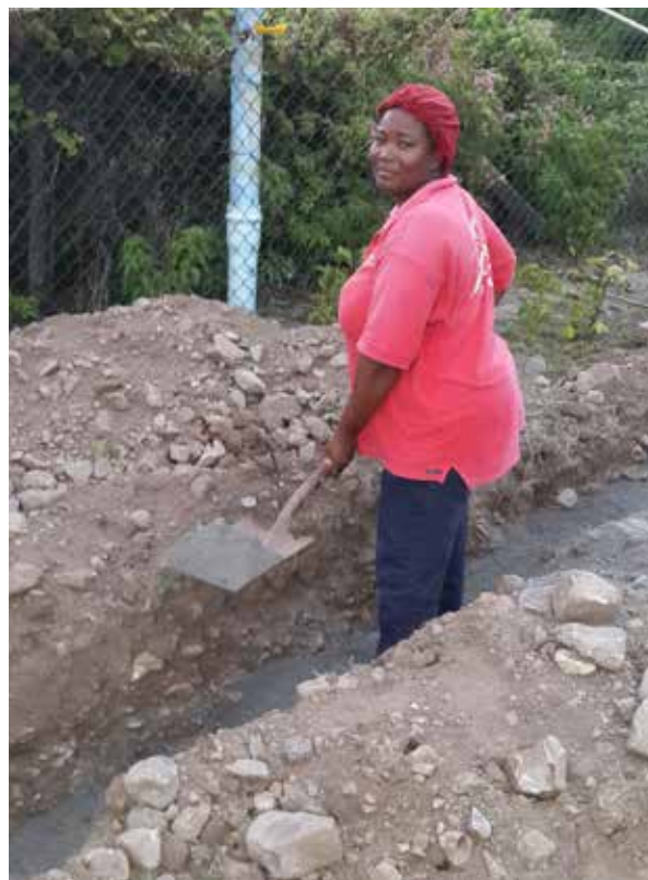
One of the Co-operative's female farmers Ms. Alana Leitch busy levelling off fill material along the trench.
