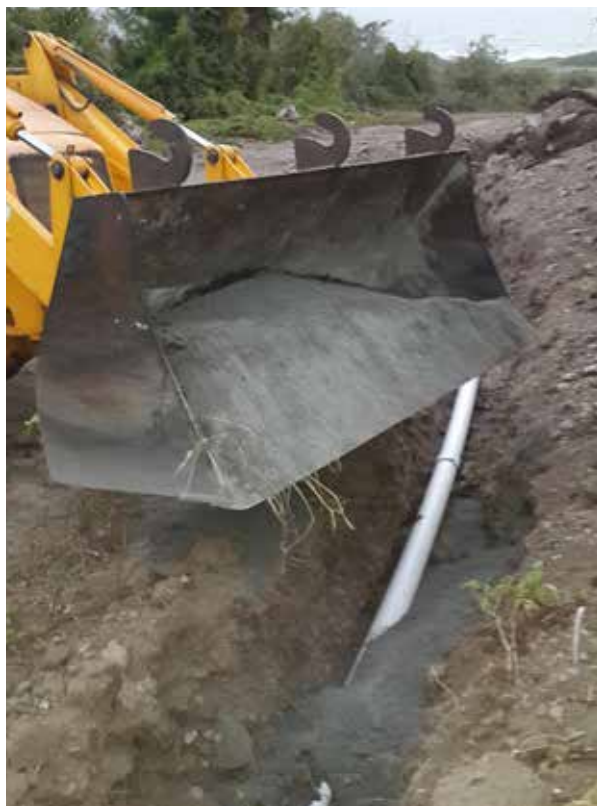
Backhoe dropping fill material to cover pipe line in the trench.
