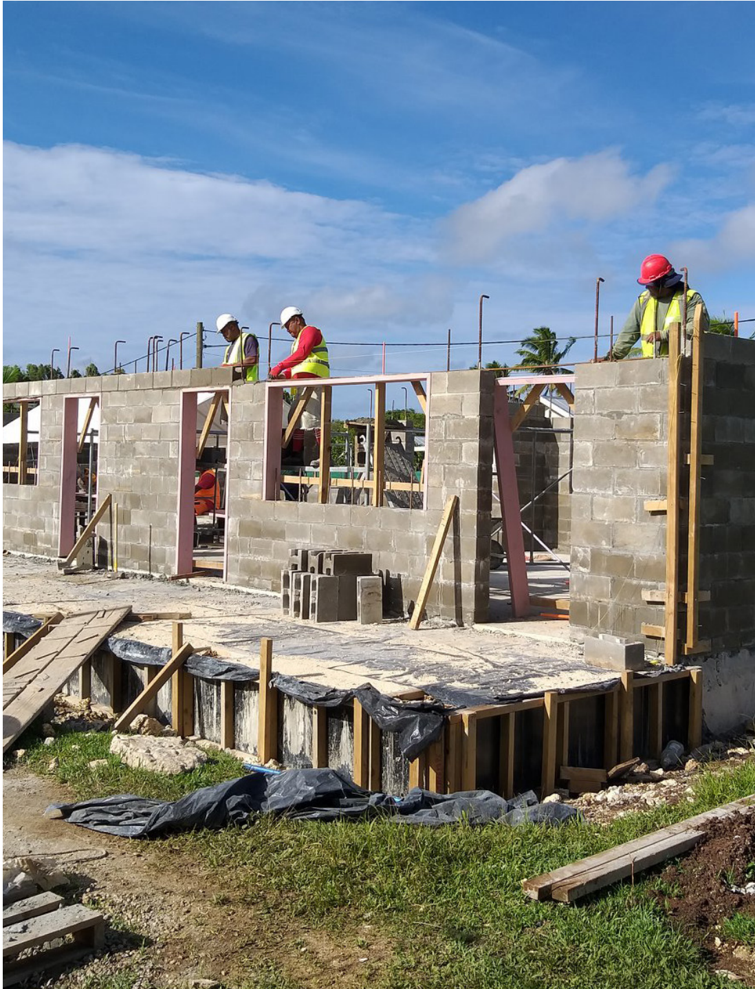
Reconstruction of Hofangahau college after Tropical Cyclone Gita (Photo: Ana Fekau Kris/PREP Tonga)
