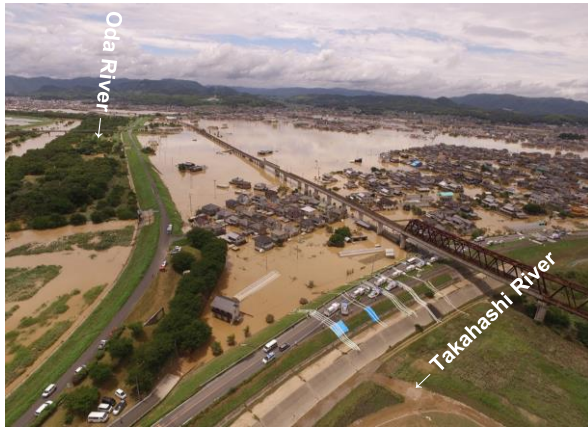
To reinforce embankments of approx. 120 rivers prone to flooding
