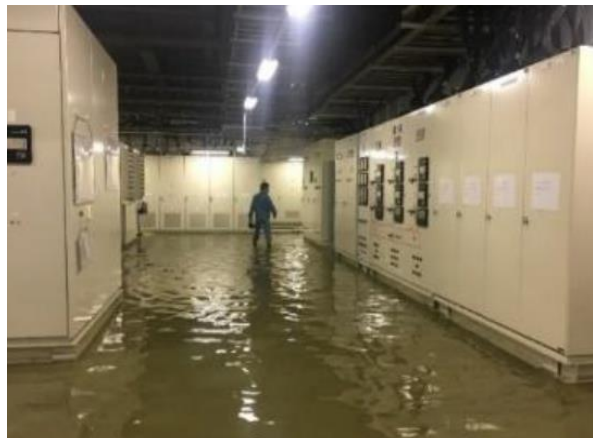
To protect the terminal buildings of 7 major airports against inundation
