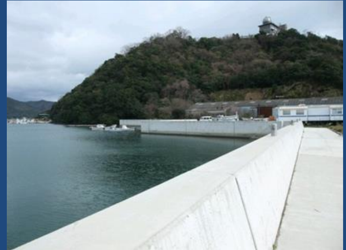
Reinforcement of tide embankment (Fukura Port)
