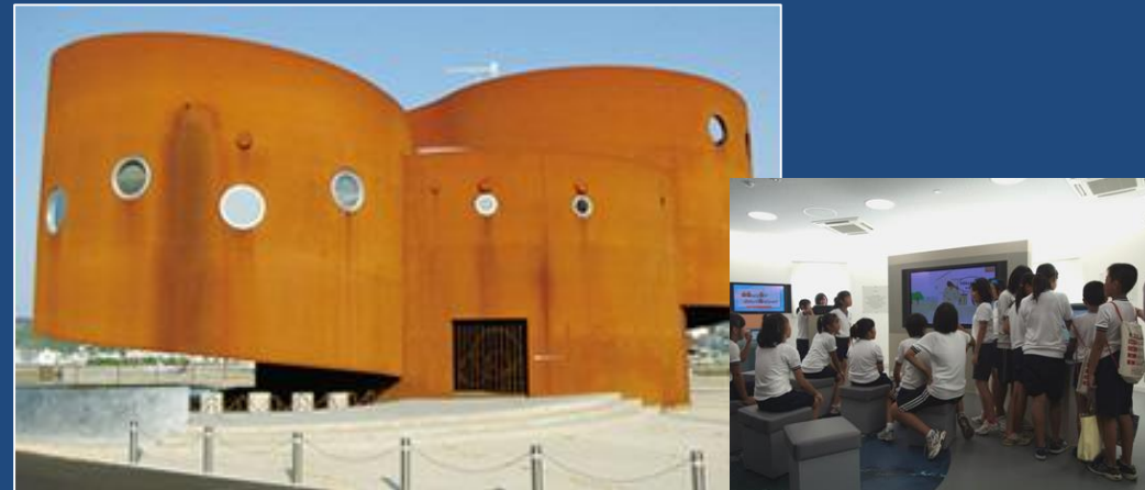
Fukura Port Tsunami Disaster Prevention Station "Uzumaru" (Disaster Prevention Learning Facility)
