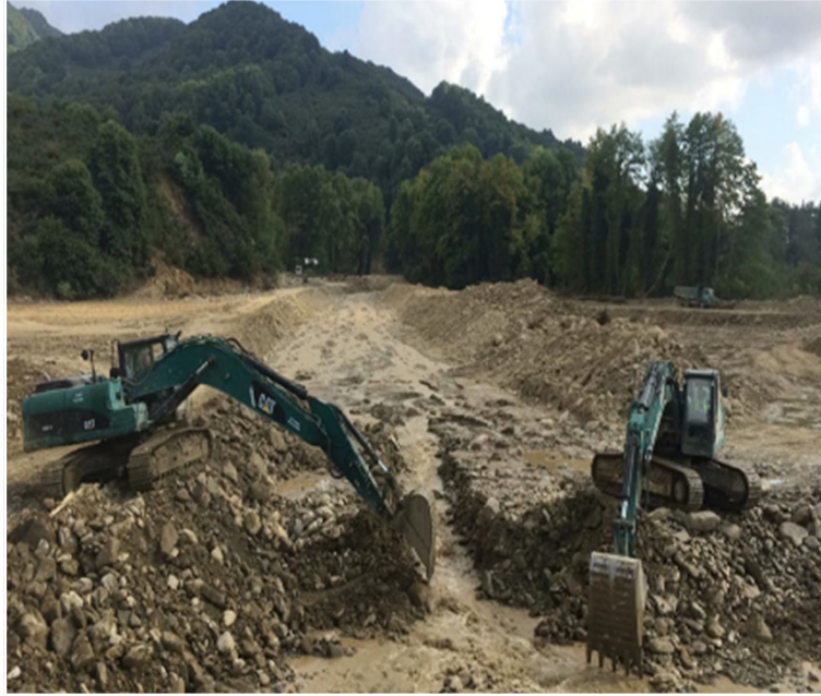
Cleaning and Expansion of Stream Beds
