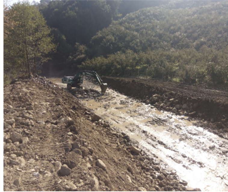
Cleaning and Expansion of Stream Beds
