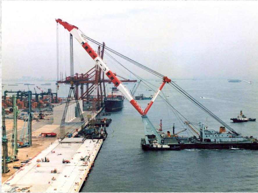
Placement Works of PC Hollow Girders
