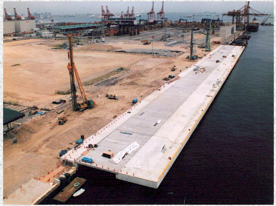
Completion of Placement Works
