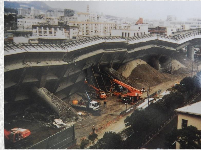
Damaged Piers of Viaduct
