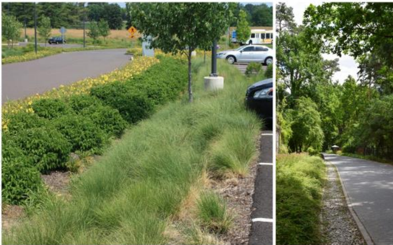
Figure 7. An infiltration trench in East Norriton, United States (left) and Podkowa Leśna, Poland (right).
