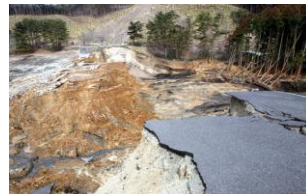
Collapsed agricultural dam, Lake Fujinuma located in the inland of the prefecture (Ebana District, Sukagawa City)
