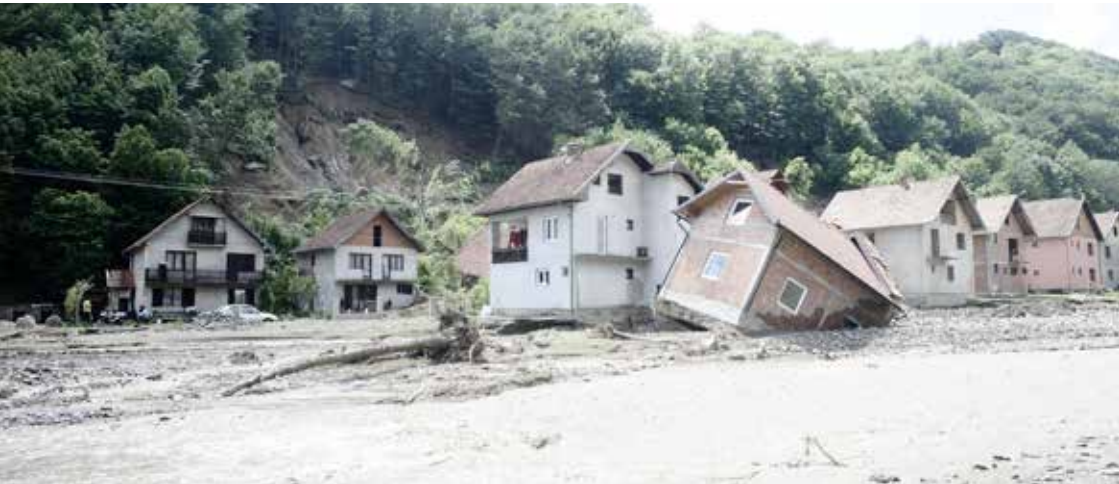
After recent heavy rains, river Cadjavica went out of stream, causing catastrophic floods and mud slides, which destroyed town of Krupanj in Macva district in central Serbia. © Dusan Milenkovic/Shutterstock
