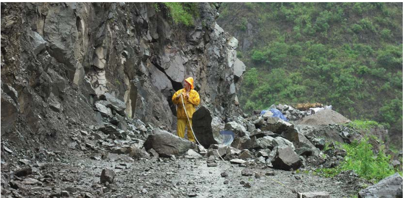
Figure 14. Measuring landslide size and intensity along recently constructed roads in the Salween River Valley Yunnan Province China © Alexia Stokes
