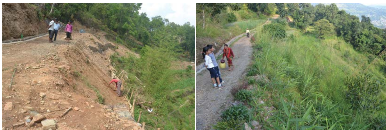
Figure 16. Demonstration site Gharelu before interventions (left) after interventions (right) (© Sanjaya Devkota)
