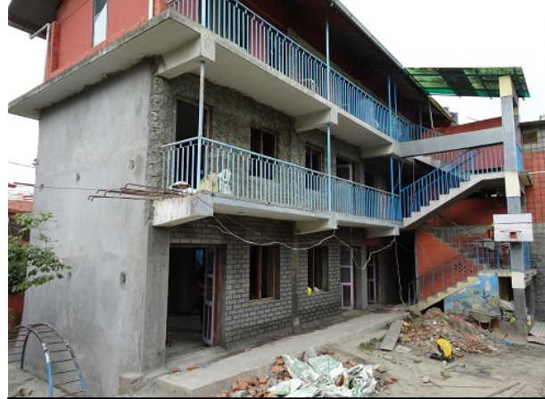
School building when the retrofitting started.
