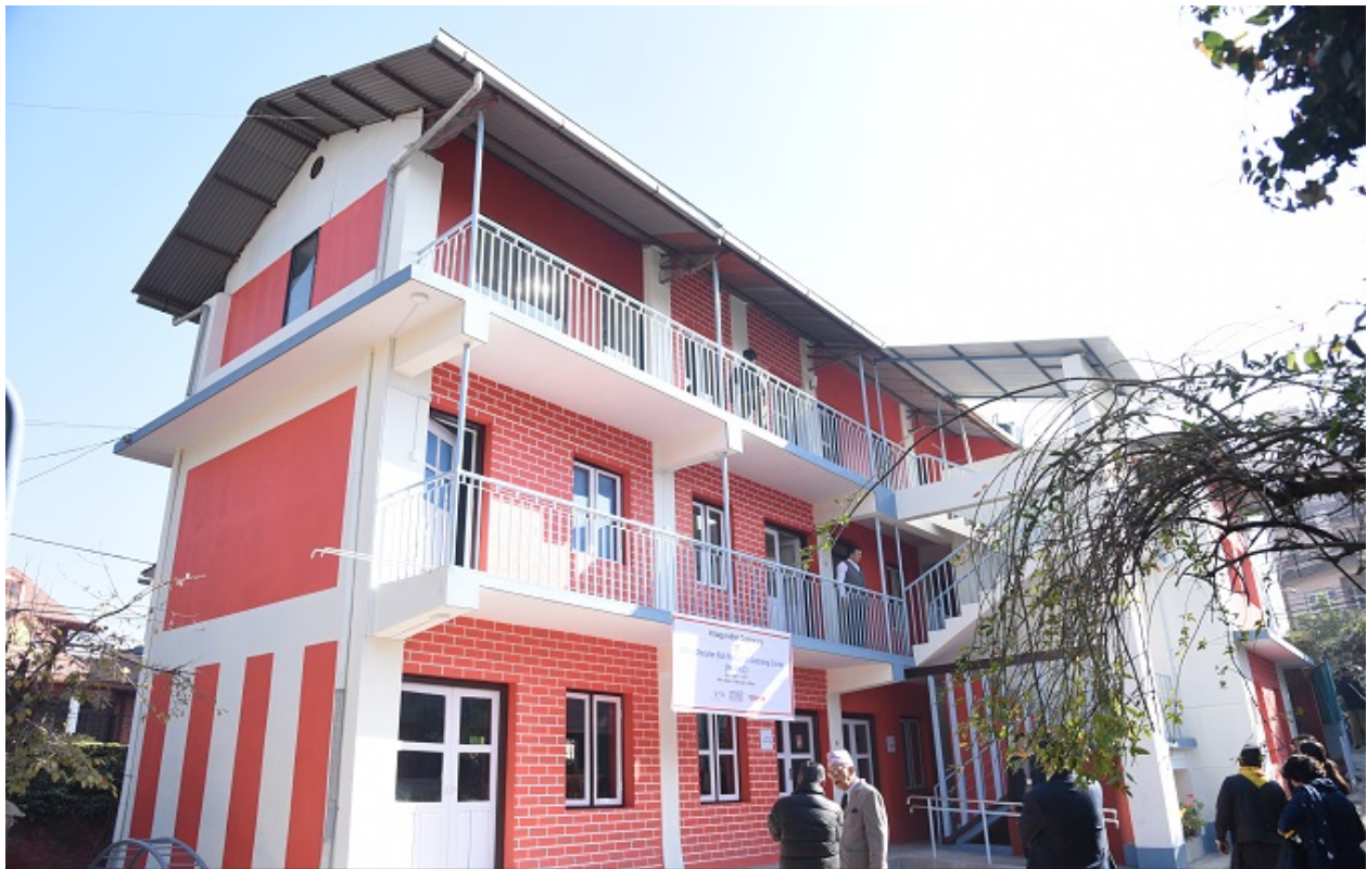
MDRRLC occupies the ground floor of the newly renovated and retrofitted building. The building also is equipped with an accessible slope with Japanese standards to make it an universally accessible building,
