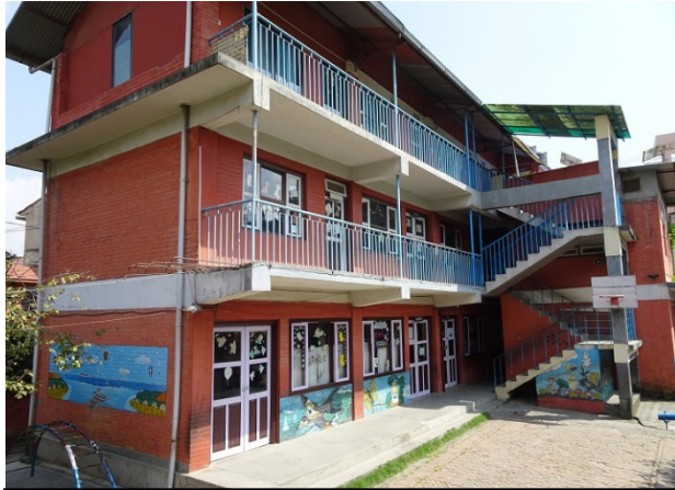
Former school building before retrofitting work.
