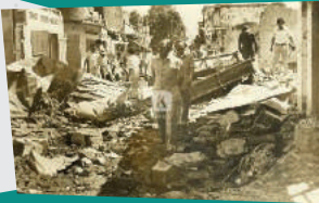
Photographs from the 1979 Lombok Island earthquake Source : Kompas
