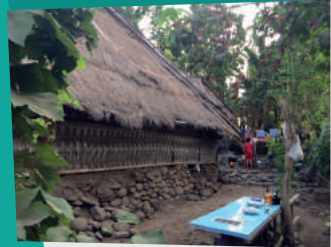
A century old earthquake-resistant traditional house in Bayan (Doc: Irina Rafliana)
